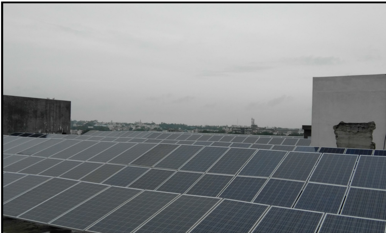
1 MW Rooftop Installation at Government General Hospital, Kurnool
